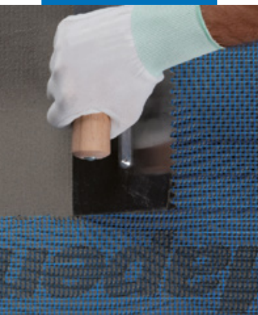
Waterproofing with Mapelastac reinforced with Mapenet 150
